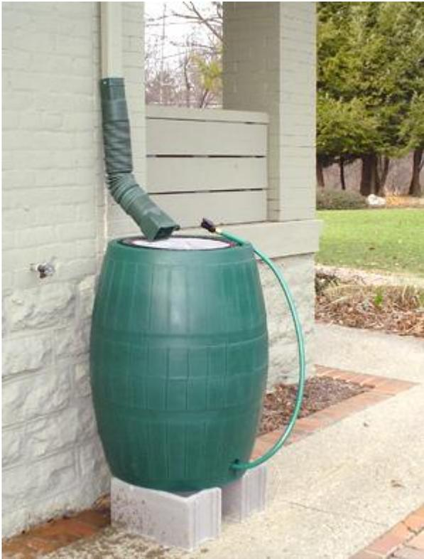
Rain barrels retain water for drier weather while avoiding erosion.
